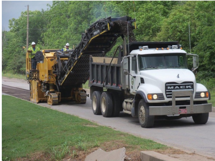
The Muscogee (Creek) Nation purchased a Volvo MT2000 milling machine to maintain roads in their Jurisdiction Area.
